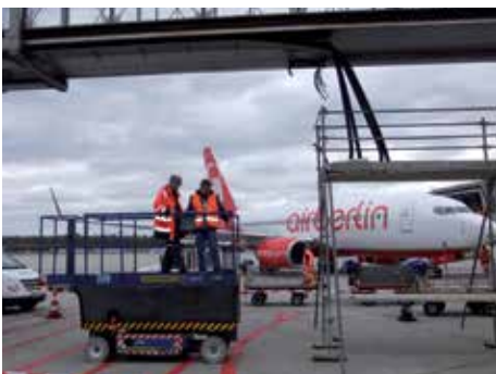
Retrofit of eight passenger boarding bridges at the Cologne Bonn Airport
