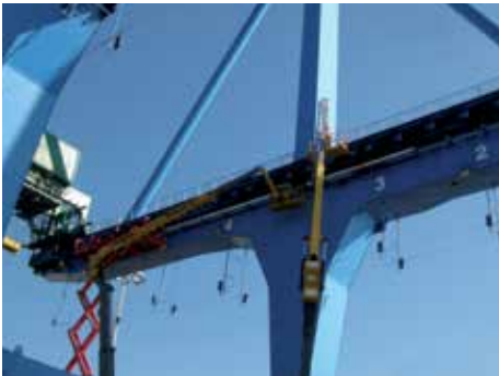
Retrofit of a festoon system to a modern e-chain system®
