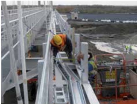
Treatment plant intake
