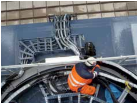
Assembly of an e-chain system® in a rotary motion
