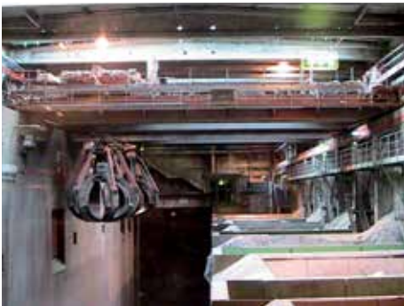
Assembly of troughs inside a bridge crane
