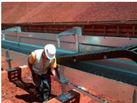
Complete installation of the e-chain®, cables, hoses, and media lines
