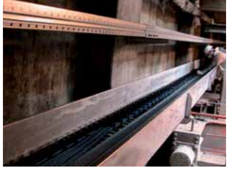
Mounting the trough along two crane bridges
